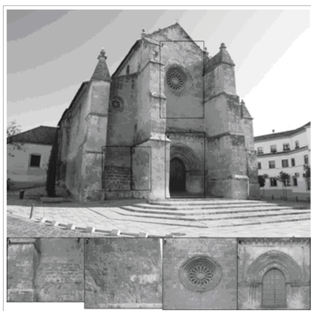
Figure 2: The Santa Marina Church, Córdoba. Insets: Areas of the building that were studied.
