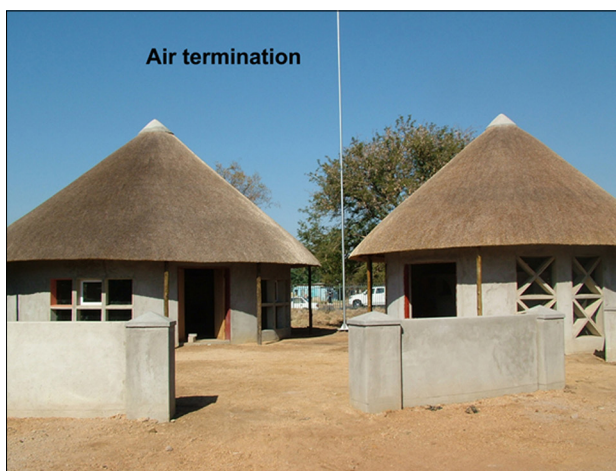
Figure 3: Thatch roof housing structures with single-mast lightning protection system.
