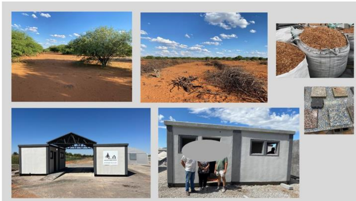
Figure 4. Clockwise from top left. Prosopis invasion in Groblershoop area illustrating absence of grass and shrubs for grazing, felled biomass, biomass chips for biomass insulated concrete construction, different aggregates in “concrete”, Prosopis biomass building in Cape Town, completed buildings made from Prosopis biomass insulated concrete at APD Upington. [Faces anonymised by journal administrator for peer review]
